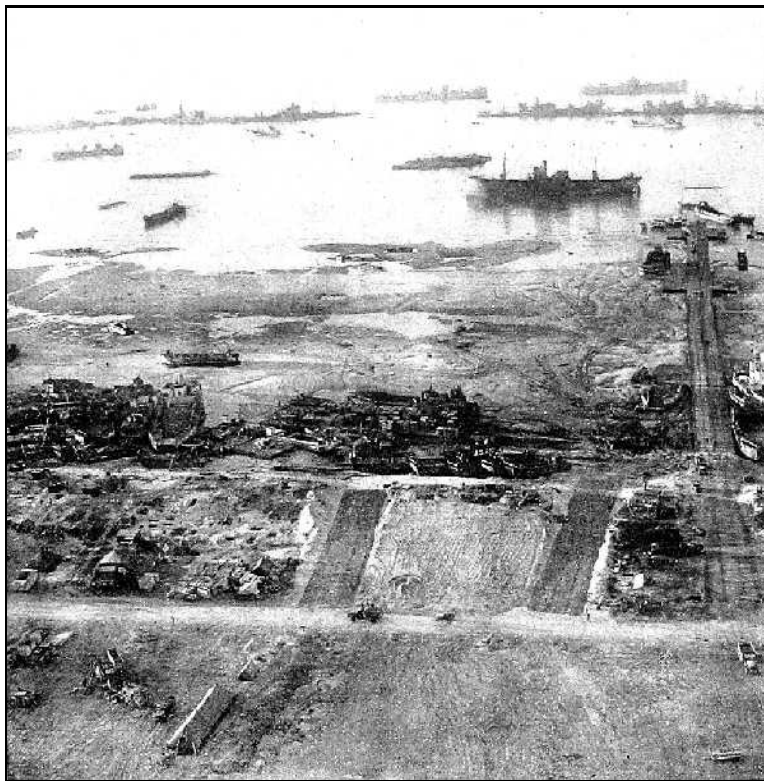
This aerial view of part of the beach area shows an artificial breakwater made of sunken ships. Other craft, "dried out" by the receding tide will float again when the water rises.
