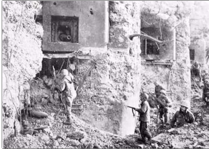
Fortifications of the Maginot Line took terrific batterings but in most cases were still useful.
