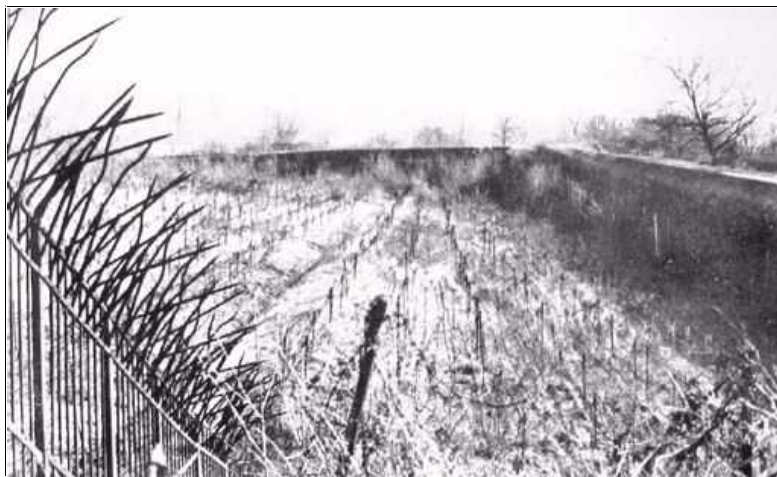
Part of the fortification and obstacles at the entrance to Fort Koenigsmacher
