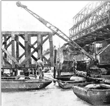
Double-triple Bailey provided permanent approach to and from Thionville.
