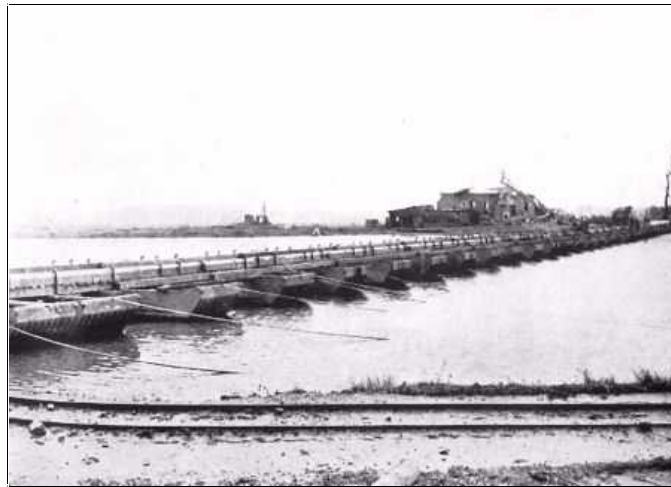
Engineer units believed this heavy pontoon bridge at Uckange (765 ft.) to be the longest in France.
