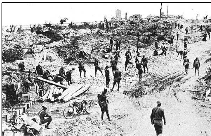
Men of the 315th Engineers and the 357th Infantry, building roads over old No Man's Land near Fey-en-Haye. The roads through Fey-en-Haye and Regnieville were obliterated by the years of artillery activity, and much work had to be done both during and after the drive, the workers being always under the eyes of enemy observers directing artillery fire.
