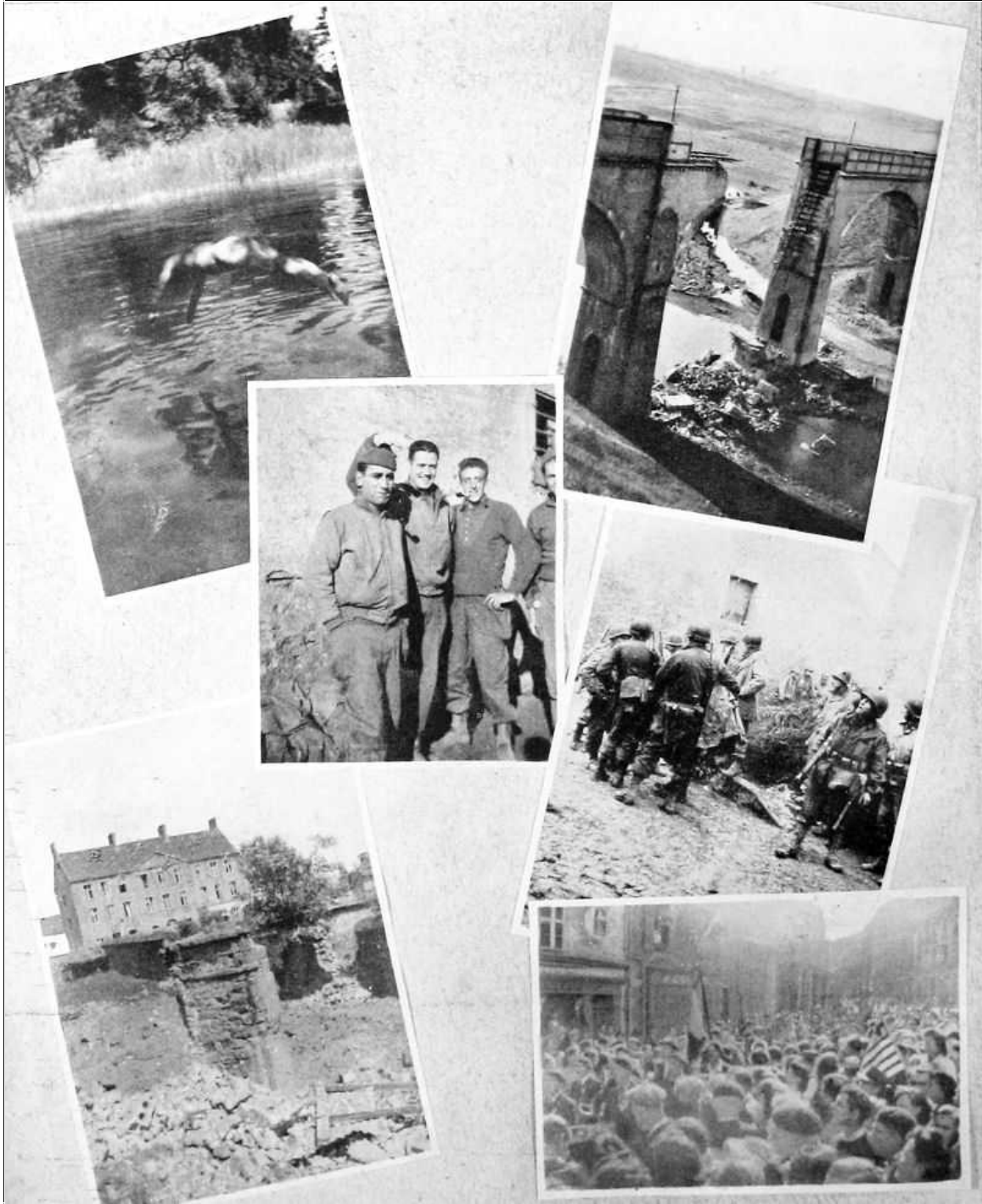
Blown bridges are encountered at Aboue in our advance toward Metz.
